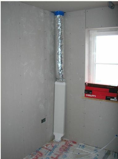
The above demonstrates a good example of how not to install. The flexible insulated duct should have been cut to the correct length so that it does not protrude through the ceiling. The flat duct would then be hidden within the partition wall, or lay flat against the partition. This would allow a shallow boxing to be formed around. Finally the Round to flat duct converters should be hidden in between joists in the floor and loft, so to create a shallower protrusion.
